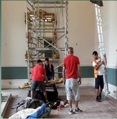
Scaffolding in the Drawing Room
